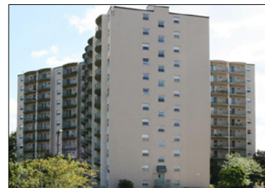
The Point at North Quincy
