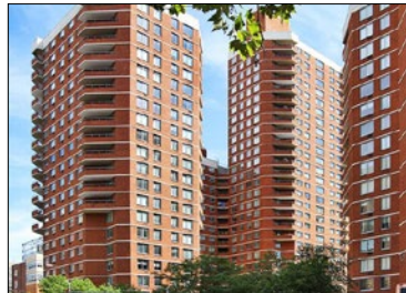
Kips Bay Court
