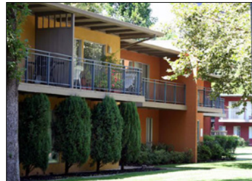
Capitol Towers and Villas
