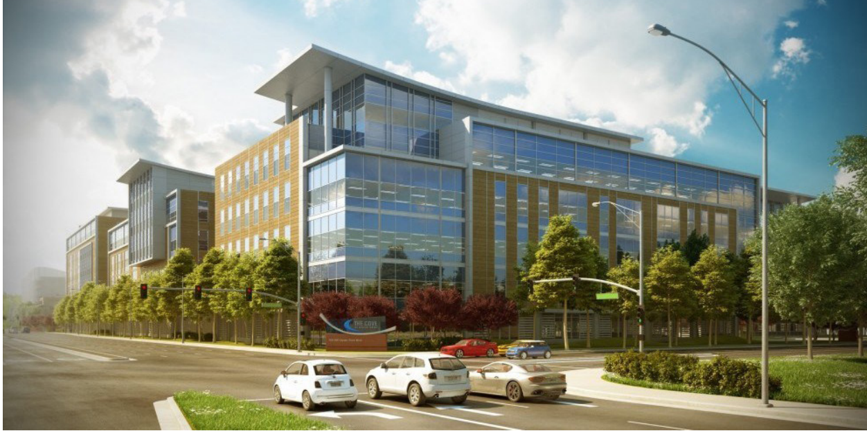
The Cove at Oyster Point, San Francisco. Rendering courtesy of Project Management Advisors Inc.
